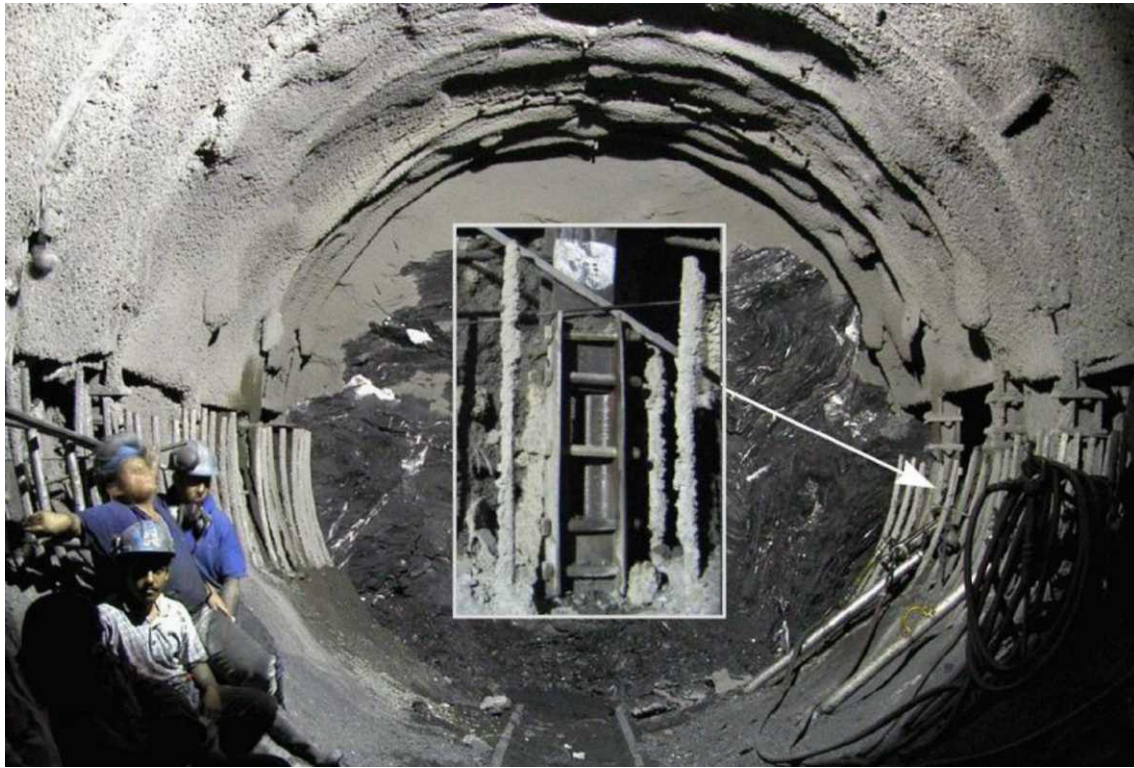
Figure 31. Initial Liner composed of circular steel arch and 20 cm of shotcrete. Inset shows detail of sliding joint with shotcrete gap. Note rebar in place to reinforce final shotcrete layer.
