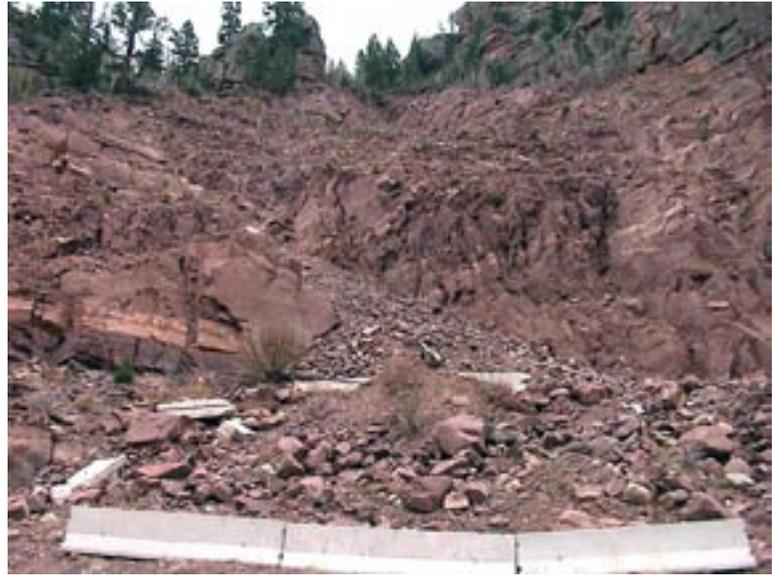
Heart of Area 1, center gully, surface roughness, planar failure.
