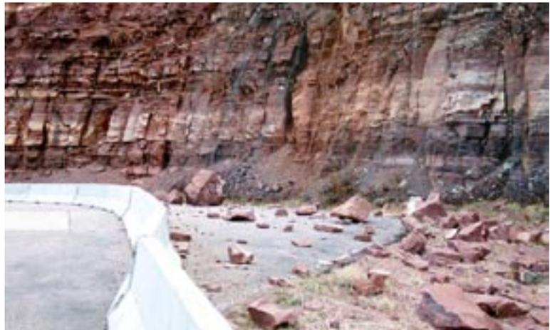
Signs of a rockfall behind the Jersey barrier. This is to be the area where the contractor will store equipment and perform work.
