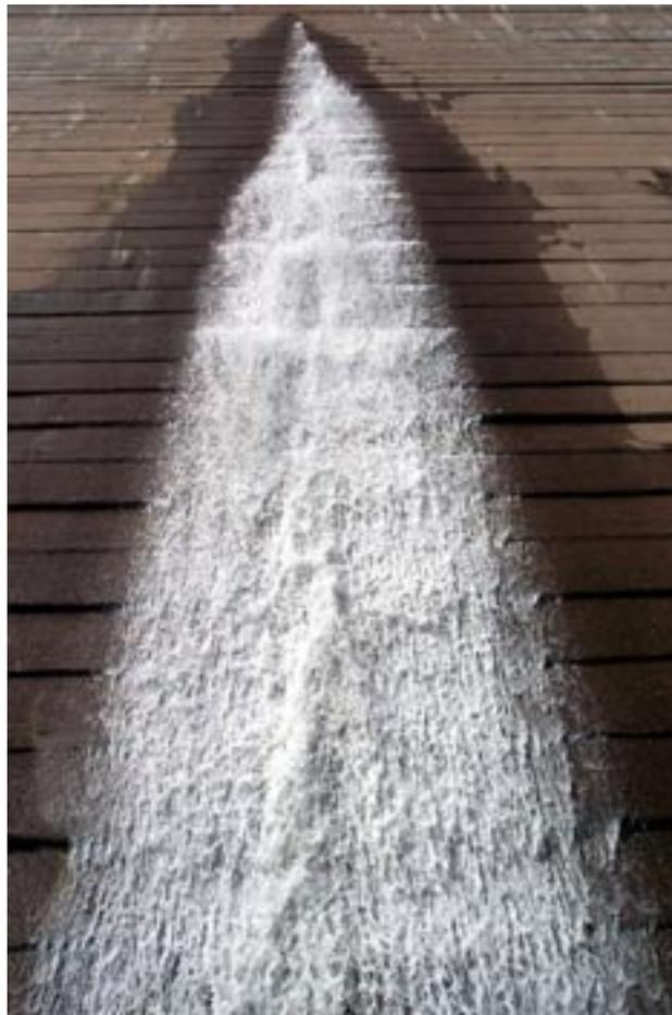
Small Inconsequential leak in the lower part of the Stillwater Dam.
