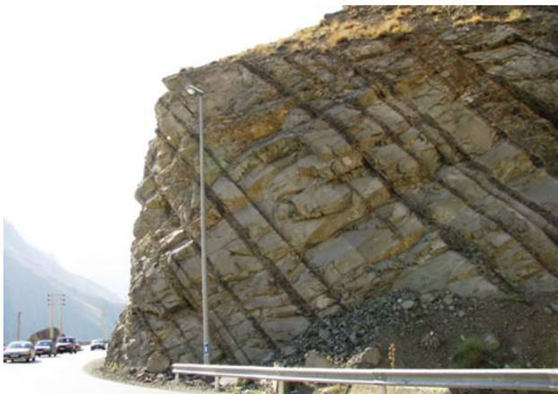
Fig. 8 Rock slope with a potential for block-flexure toppling failure facing Chalus Road
