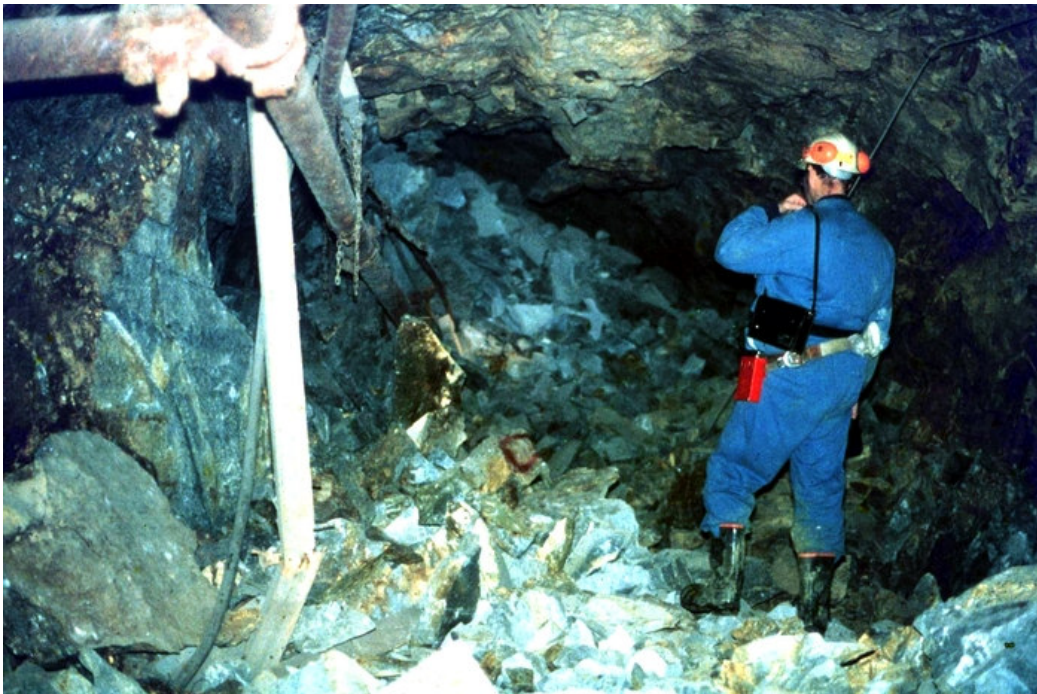
Figure 3: Results of a rockburst resulting from the collapse of a pillar in an underground mine.
