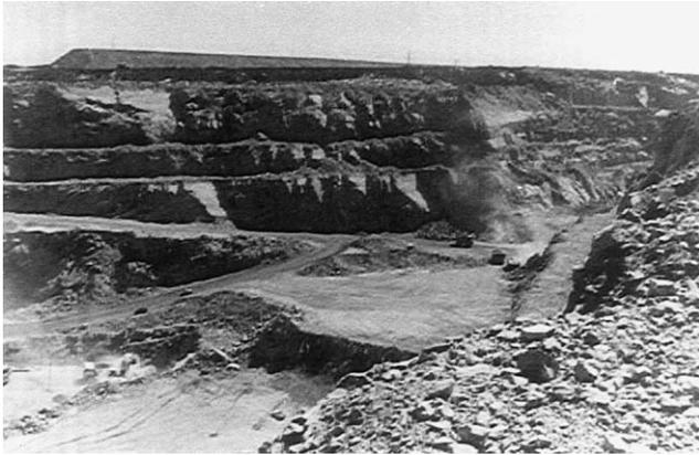
Fig. 9. Planar failures on the western highwall.
