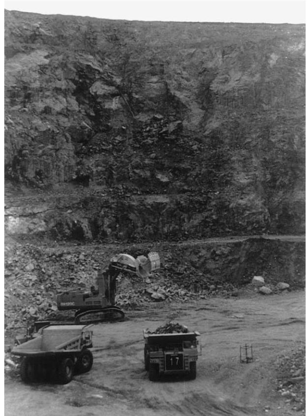
Fig. 14. Circular failure on the south-east highwall of the satellite pit.
