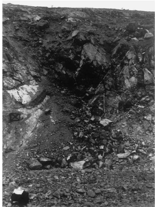
Fig. 12. An example of a small wedge failure.
