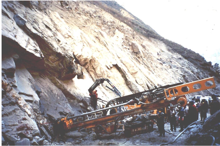
Figure 16: Drilling machine for the installation of 40 m long reinforcing cables in 150 mm diameter holes in a dam excavation.
