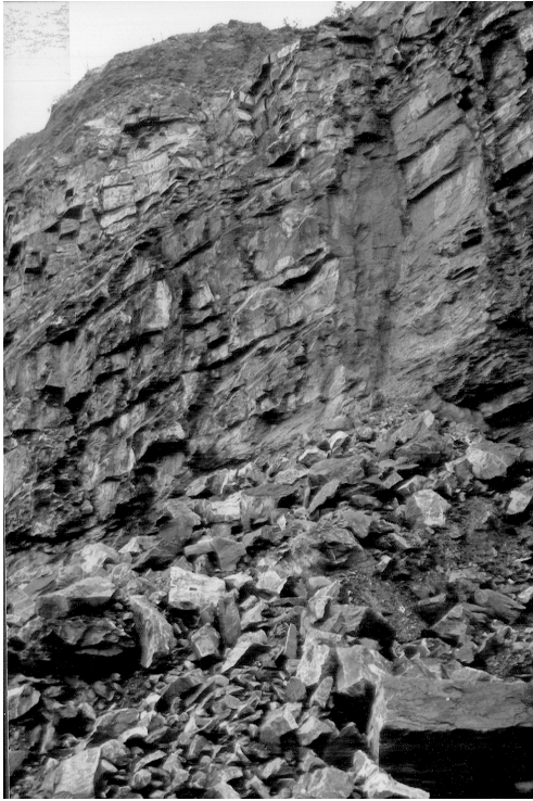
Fig. 23. Structurally controlled failure in the face of a steep bench in a heavily jointed rock mass.
