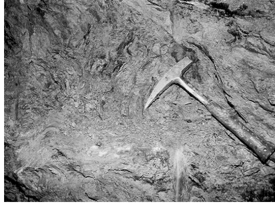
Fig.20. Appearance of the very poor quality Athenian schist at the face of the side heading illustrated in Fig. 19.
