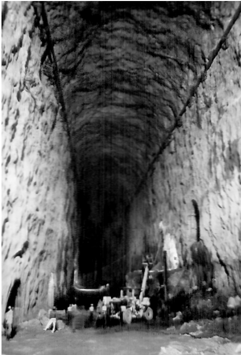
Fig. 14. Partially completed 20 m span, 42.5 m high underground powerhouse cavern of the Nathpa Jhakri Hydroelectric project in Himachel Pradesh in India. The cavern is approximately 300 m below the surface.
