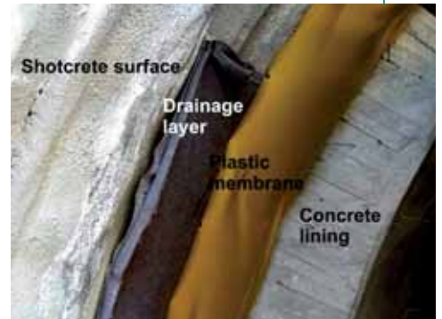
Below: drainage and waterproofing layers behind the concrete lining.
