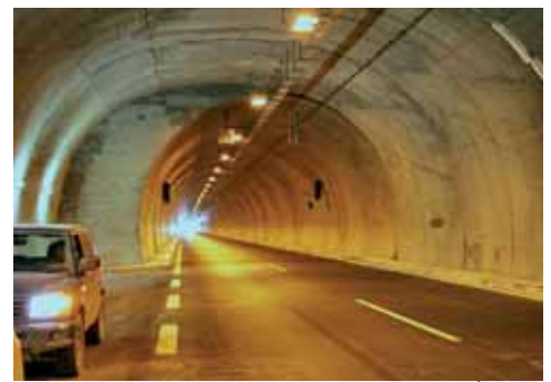
Above: a parking bay in a typical operating tunnel on the Egnatia highway
