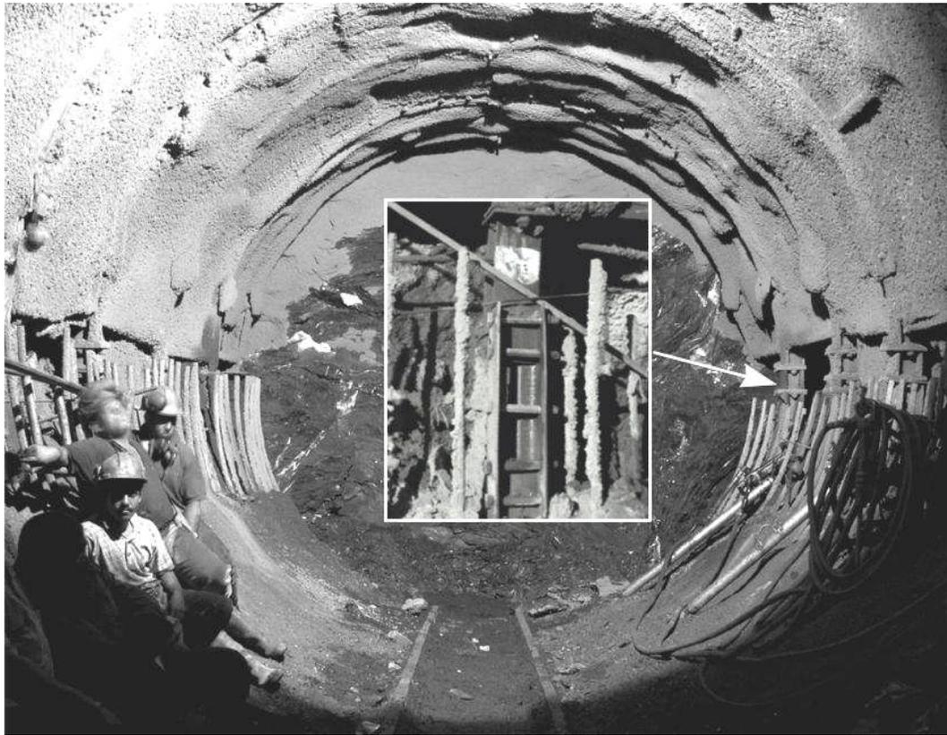
Figure 31. Initial Liner composed of circular steel arch and 20 cm of shotcrete. Inset shows detail of sliding joint with shotcrete gap. Note rebar in place to reinforce final shotcrete layer.
