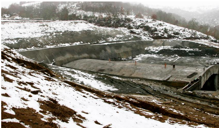
Figure 22. Kiloma tunnel exit portal in molassic rocks showing cover and cut construction and small surficial slide on the left hand side of the photograph. The cover and cut structure protected the portal from further development of this slide.
