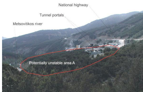
Figure 7: Potential instability in area that will be crossed by the Egnatia highway under the national highway. The portals of tunnel indicate the alignment of the Egnatia highway.
