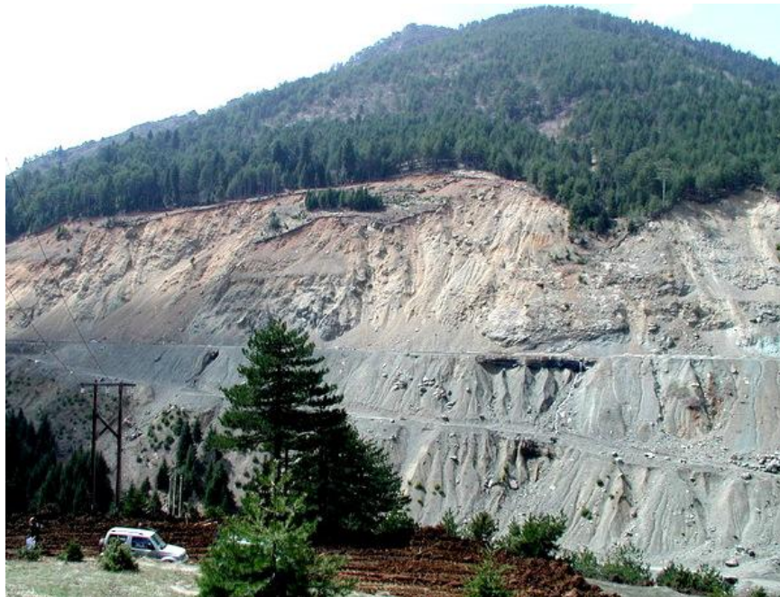
Figure 23 General appearance of Big Cut with the Egnatia Highway platform running across the centre of the picture. The slope is a peridotite with disordered serpentinisation and tectonic shearing
