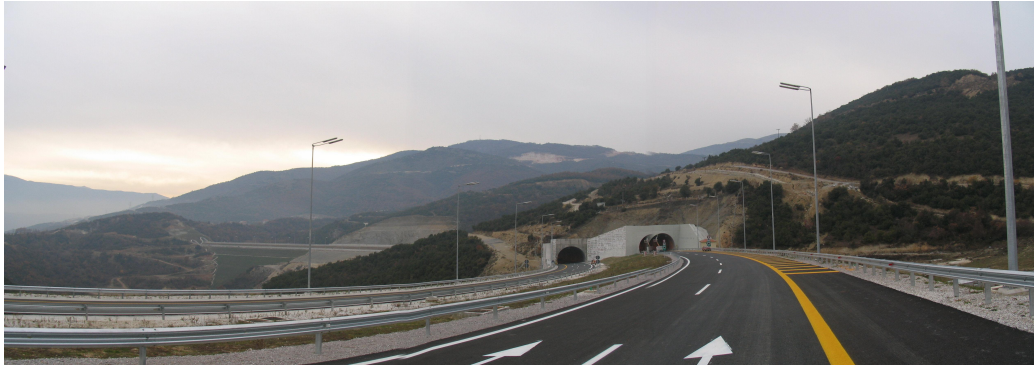
Figure 10. The tunnel S3 in the central part of the highway from the entrance portal, crossing an unstable slope stabilized during the construction
