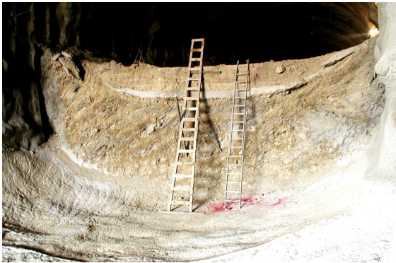
Figure 11: Appearance of the phyllitic formation in the face of the remaining bench of tunnel S3. The well preserved structure of the rock mass is clearly visible in this face.
