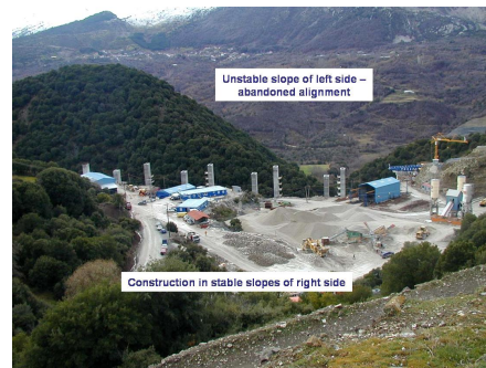
Figure 4 Construction works at the north side of Metsovitikos valley after the realignment of the highway in the Metsovo section in order to avoid globally unstable slopes at the south side of the valley
