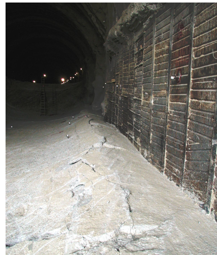
Figure 12: Severe invert cracking near the entrance portal of the S3 tunnel.
