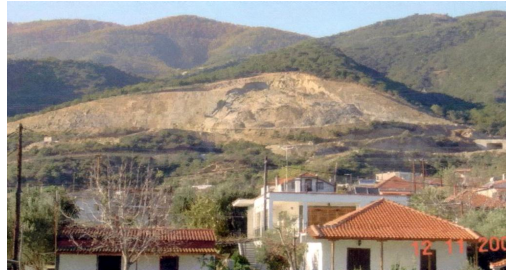
Figure 21. The landslide of figure 20. the rotational failure is clear
