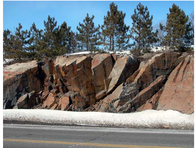
Fig. 14. Road cut in which the size of individual rock blocks is of the same order as the height of the cut. Rock mass classifications, based on the assumption of homogeneity, cannot be applied to this rock mass.
