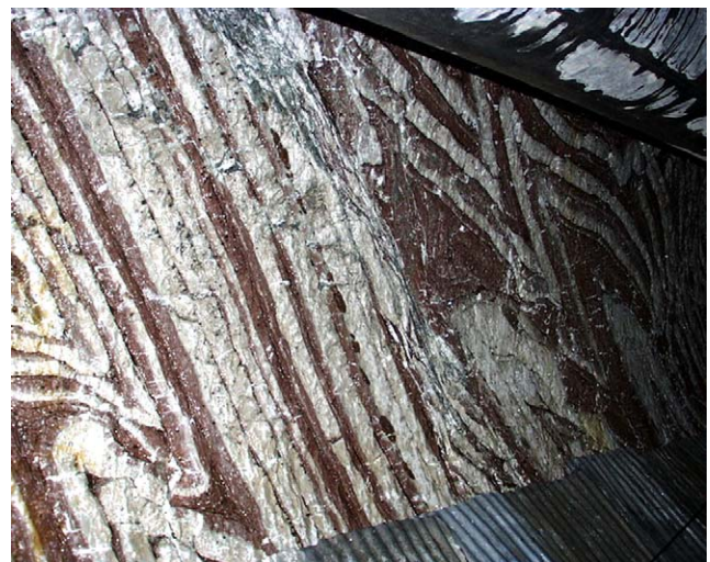
Fig. 20. Undisturbed conditions achieved by TBM excavation in folded sedimentary rocks in the Acheloos tunnel in Greece.
