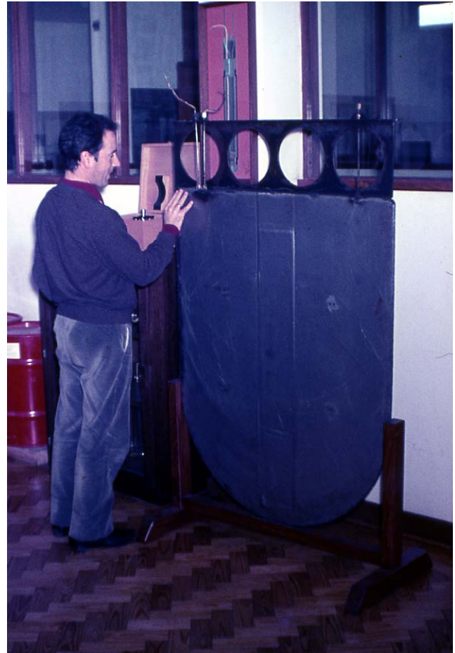
Fig. 6. Flat jack for installation in the deep slot created by the saw shown in Fig. 5. Photographed by E. Hoek in LNEC laboratory, Lisbon, 1974.
