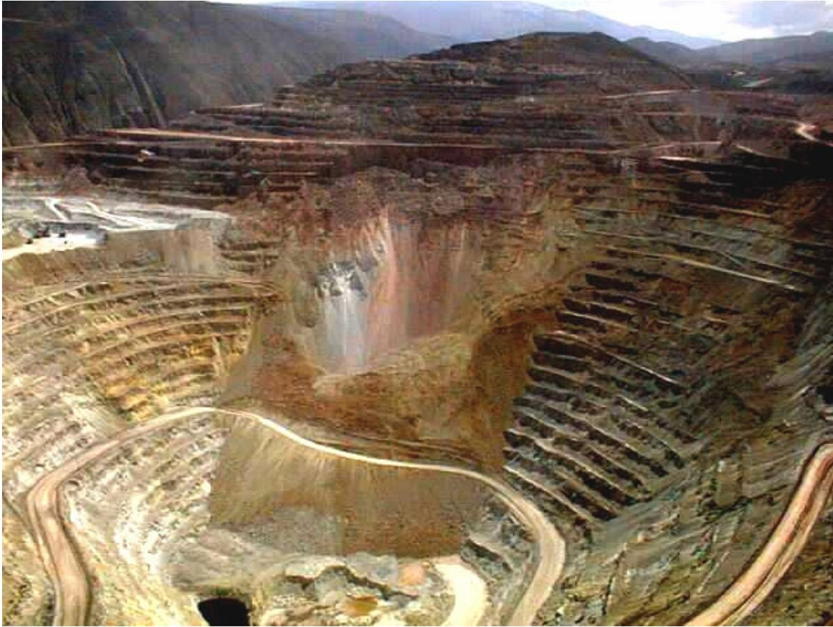
Figure 2: A large scale slope failure in an open pit mine.
