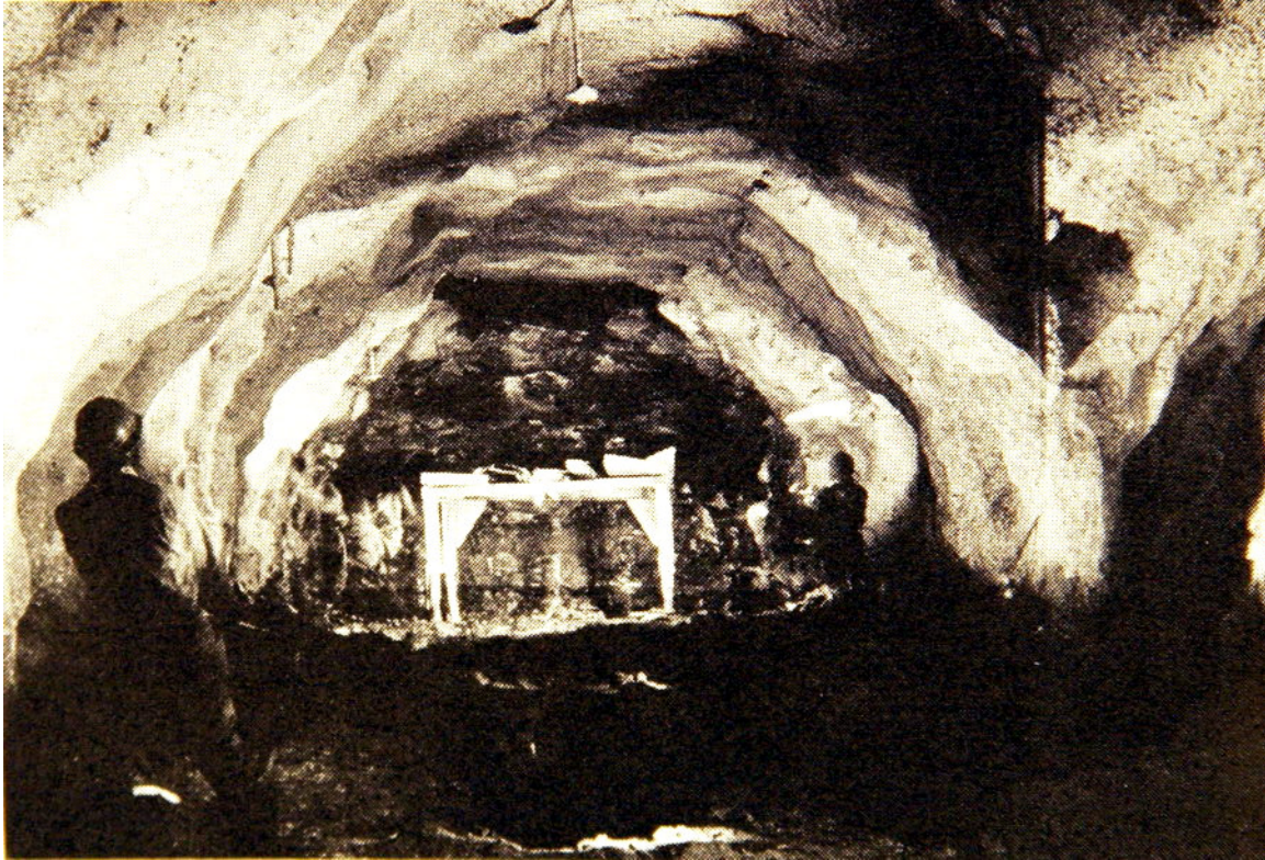
Figure 14. Penstock test chamber – excavation of upper bench
