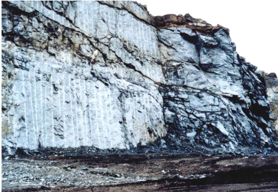
Figure 1: Comparison between the results achieved by pre-split blasting (on the left) and normal bulk blasting for a surface excavation in gneiss.
