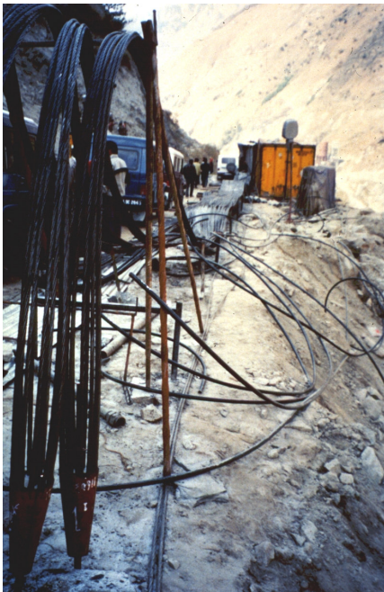
Figure 16: Drilling machine for the installation of 40 m long reinforcing cables in 150 mm diameter holes in a dam excavation.
